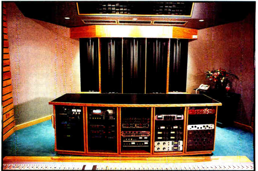
Custom RPG diffuser system in Caracole's control room
