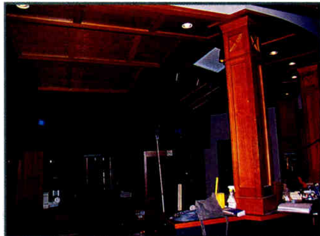
Wood control room (under construction) at Armoury Studios
