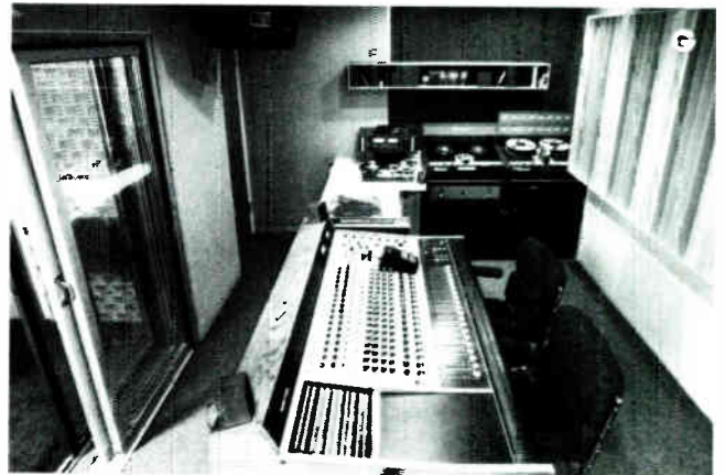
G. Soundwave, a facility in Washington, DC, recently underwent a major overhaul of its Studio C. Renovations were handled by Chips Davis LEDE Designs and included the installation of a new front shell covered with absorptive Armstrong Soundsoak 85, RPG Diffuser panels to the rear of the NEOTEK Series II console, UREI 809 monitors and Crown Micro-tech 1200 amplifiers. The 16-track studio is primarily used for video sweetening and soundtrack work.
