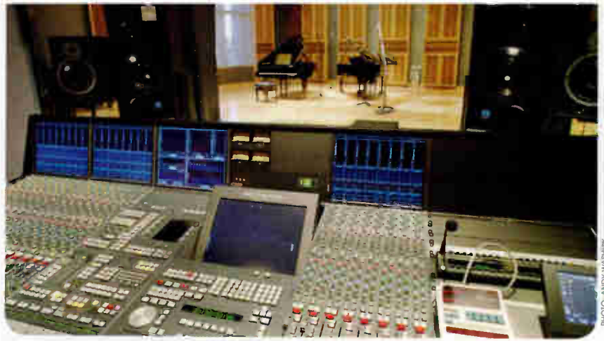
Radio control room A at WGBH Boston has an SSL C200 console.
