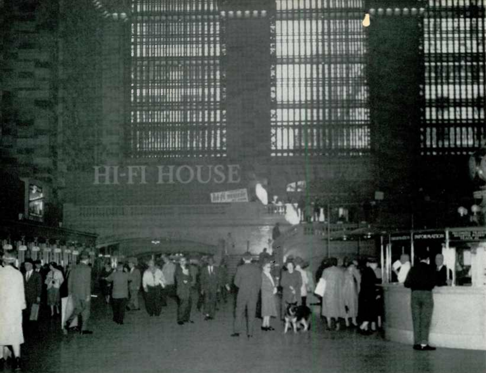
At the Vanderbilt Avenue balcony of New York's Grand Central Station, Hi-Fi House vies for attention with the famous Kodak sign at the opposite end of the upper level. Below, Hi-Fi House looked like this when it was under construction, with the steel framework completed
