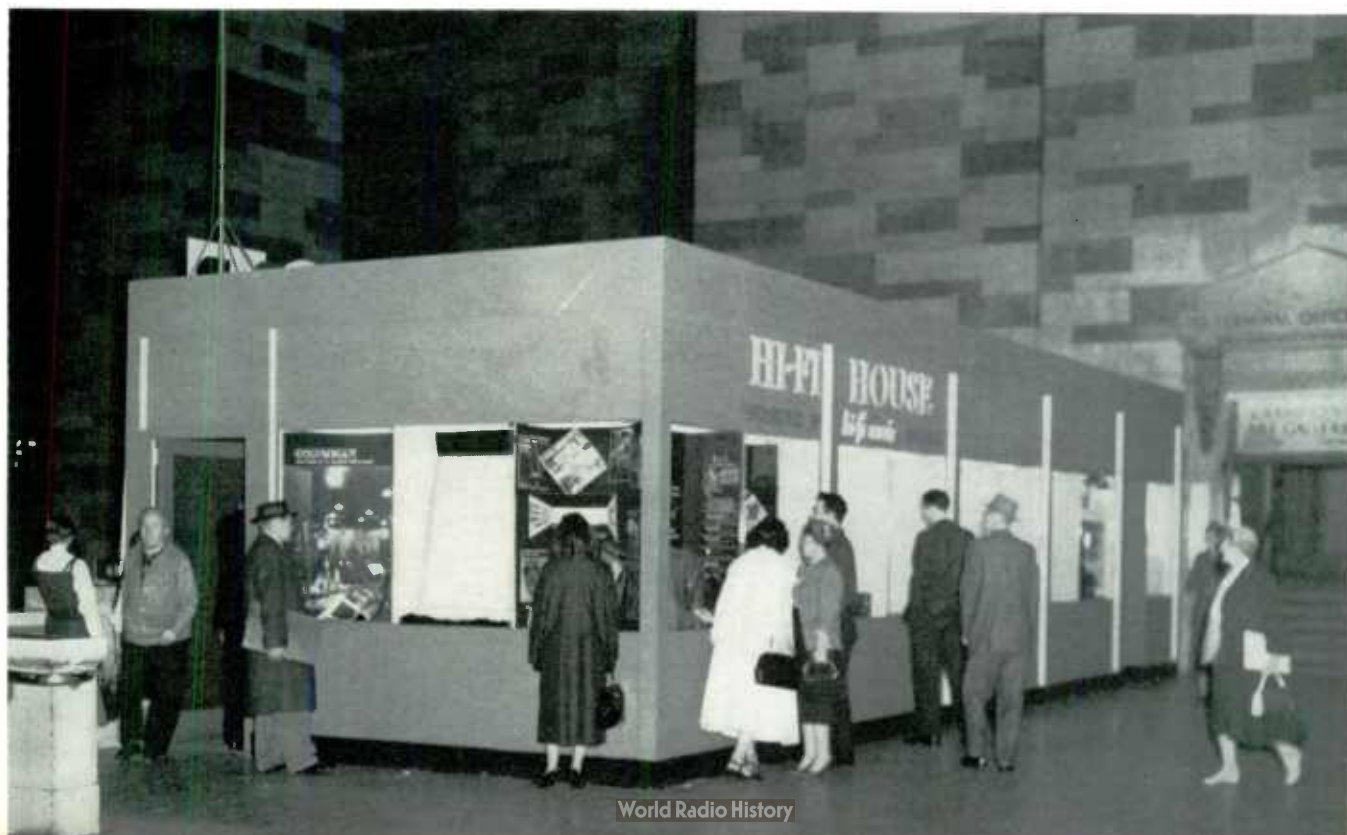
The front door is between the broad marble stairs, left, and the Vanderbilt Avenue entrance to the Terminal. Exit door is at the far right
