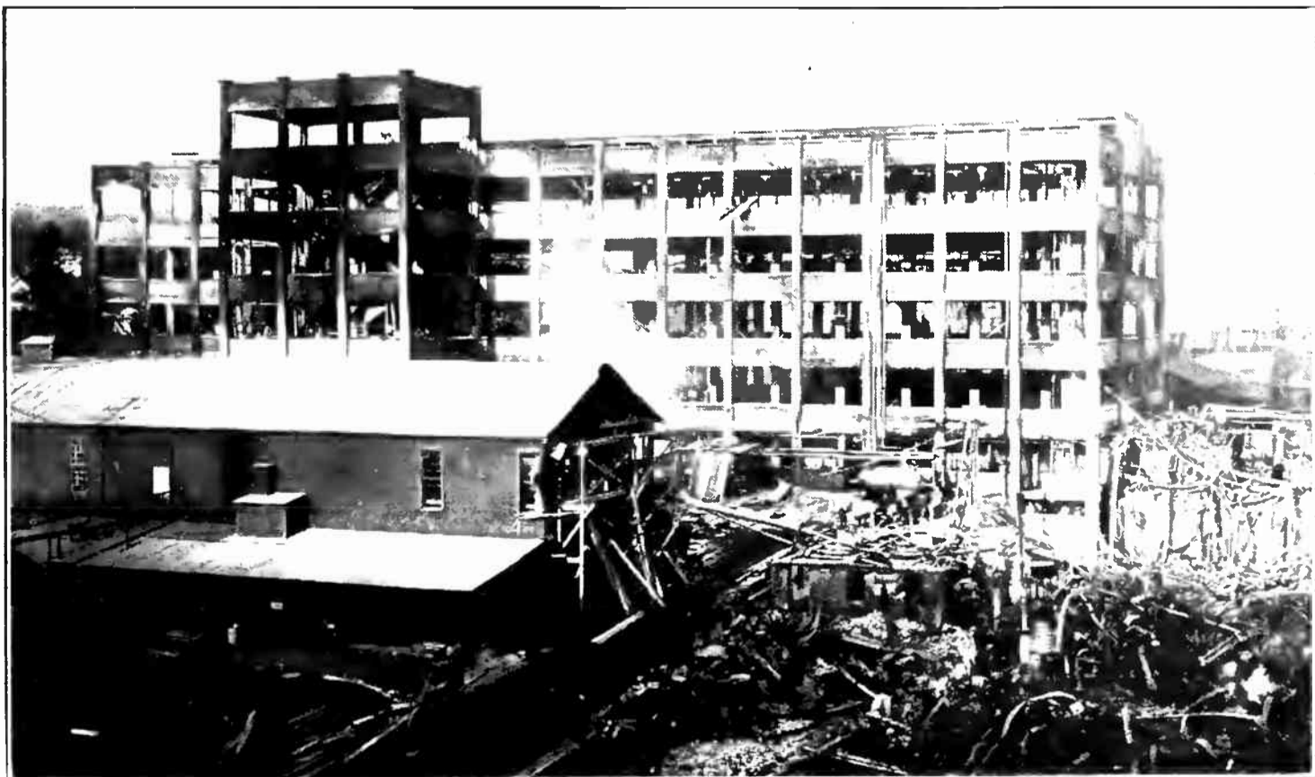
No. 24 Building, the huge Record Making Plant, looking North. Both Blue Amberol and Disc Records were manufactured here.
