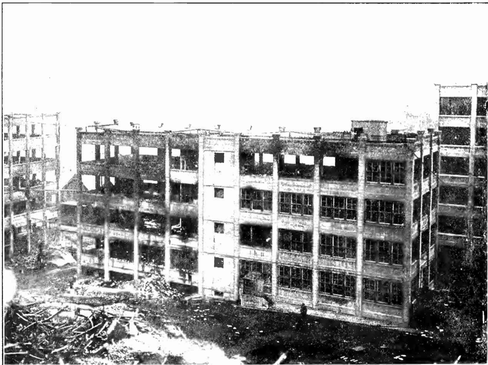
North side of the Administration Building, looking south. Right hand end is where fire was checked before reaching the Laboratory adjoining. Storage Battery Building appears on the right.
