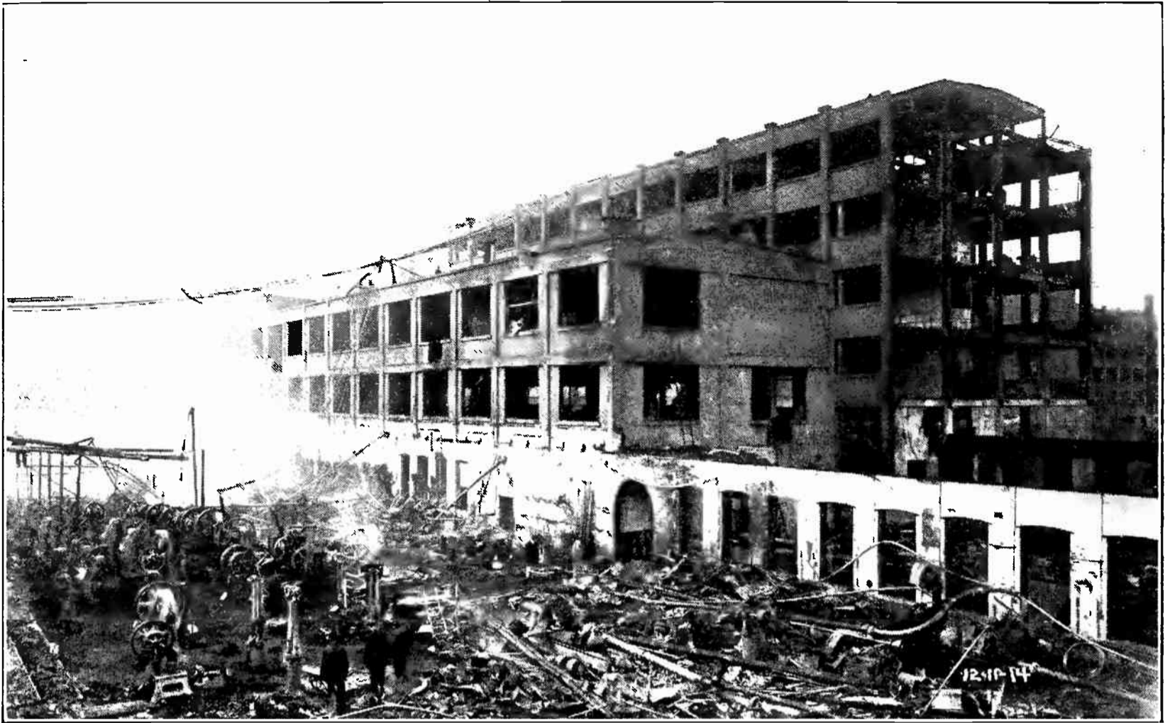
Looking South. Buildings Nos. 11 and 13 with remains of Punch Press Dept. in foreground. Total Loss.
