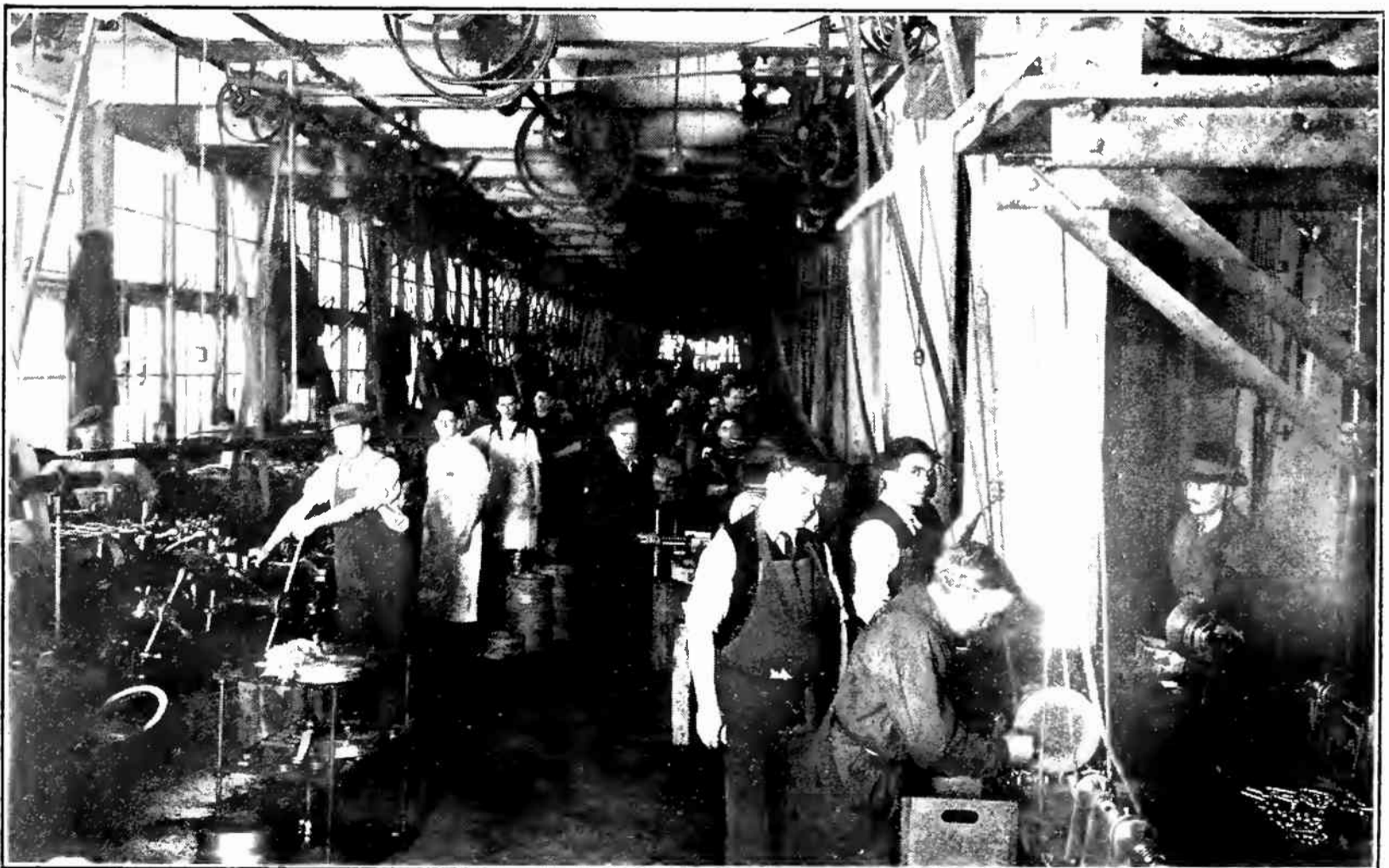
SCREW DEPARTMENT, STORAGE BATTERY BUILDING
