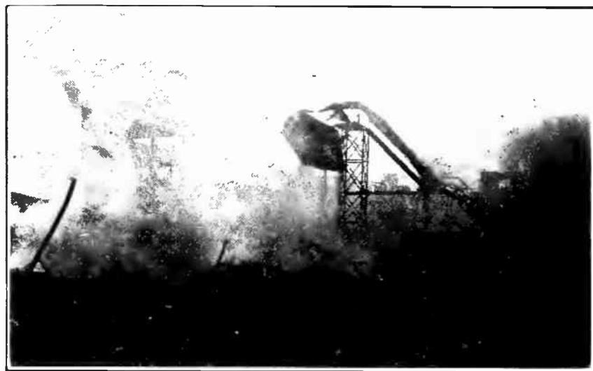
Remains of Dust Collector in Cabinet Shop.
