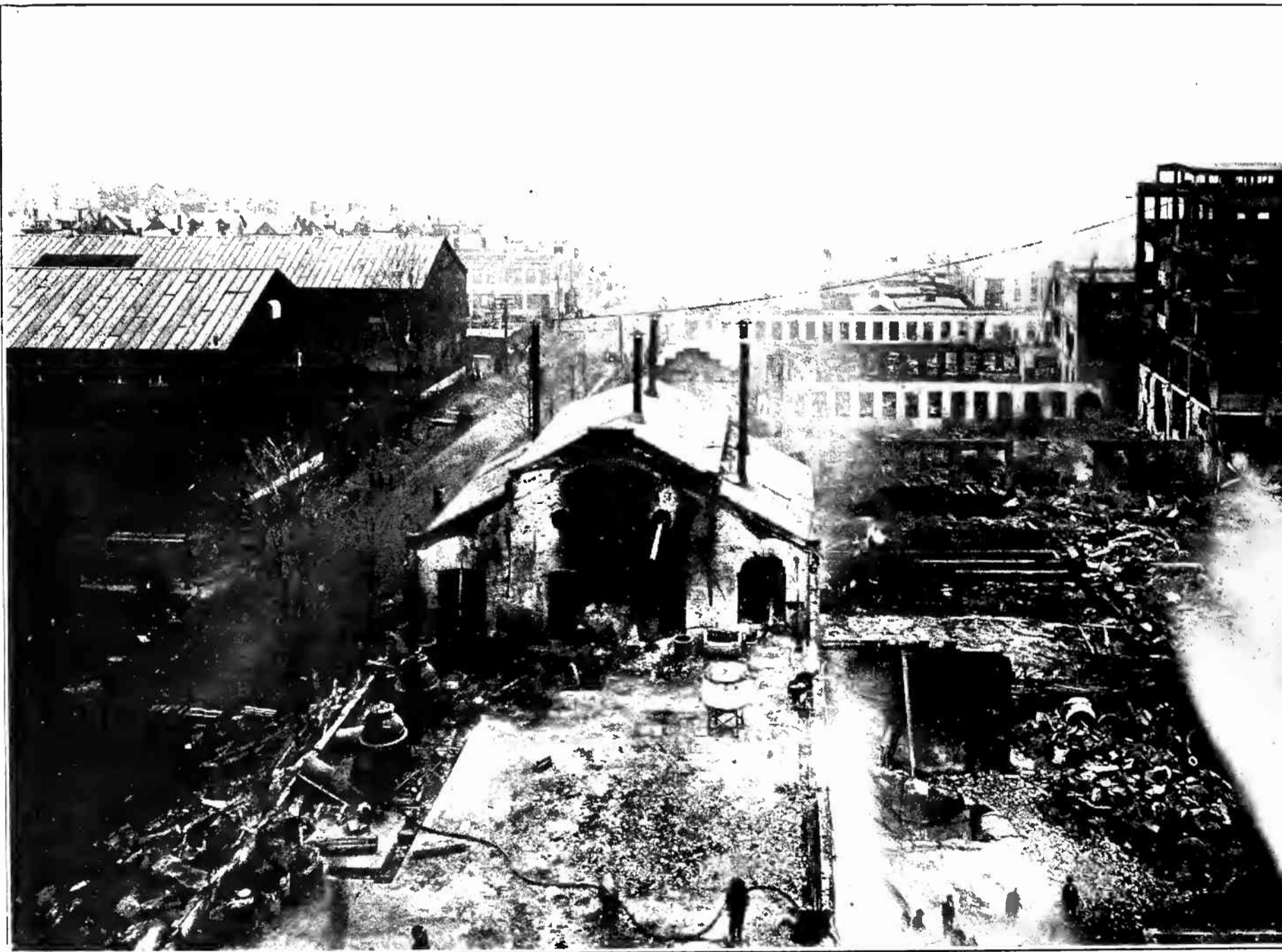
GENERAL VIEW C
