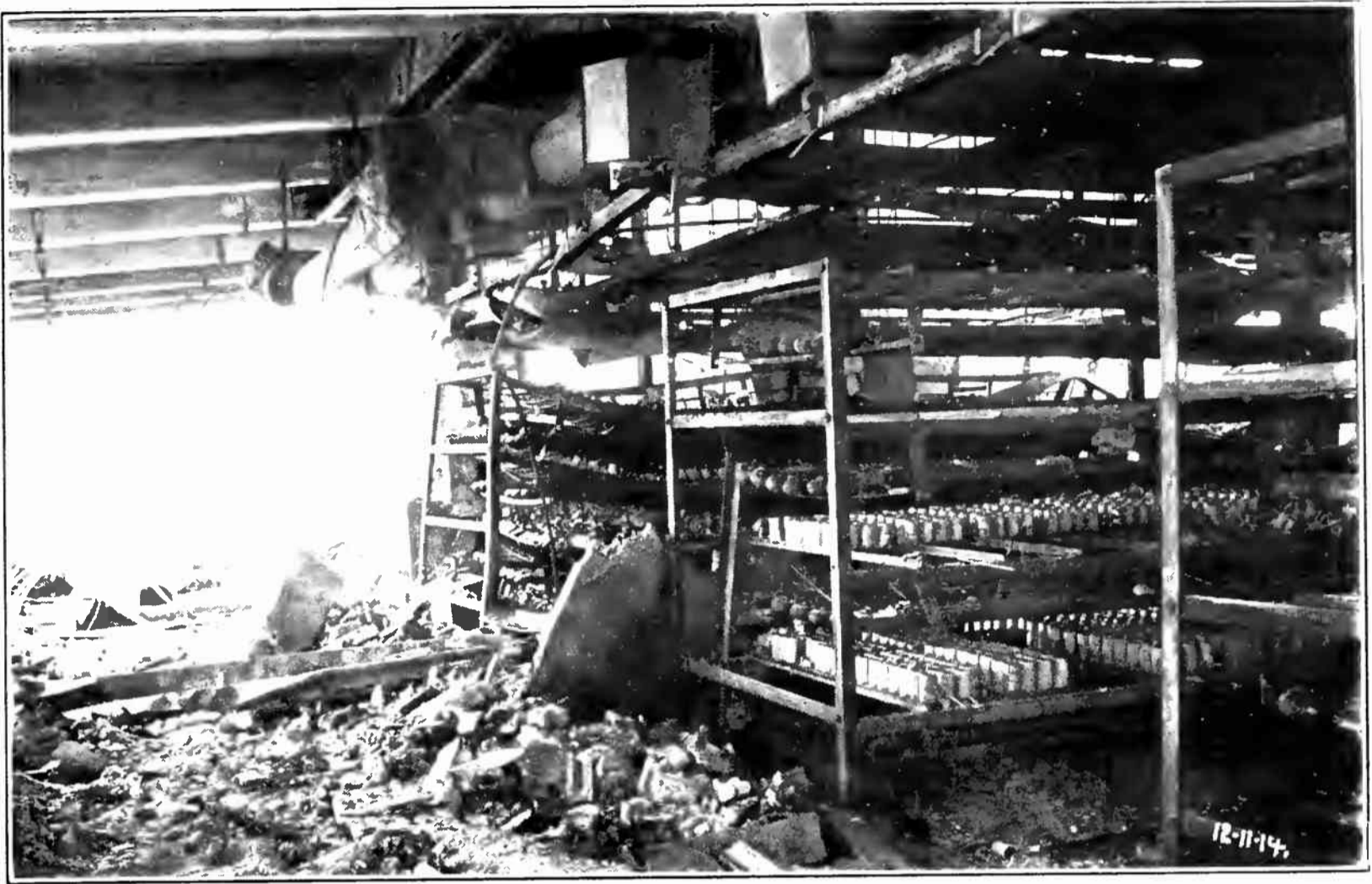
Remains of Blue Amberol Drying Ovens in north end of Building No. 24, top floor.
