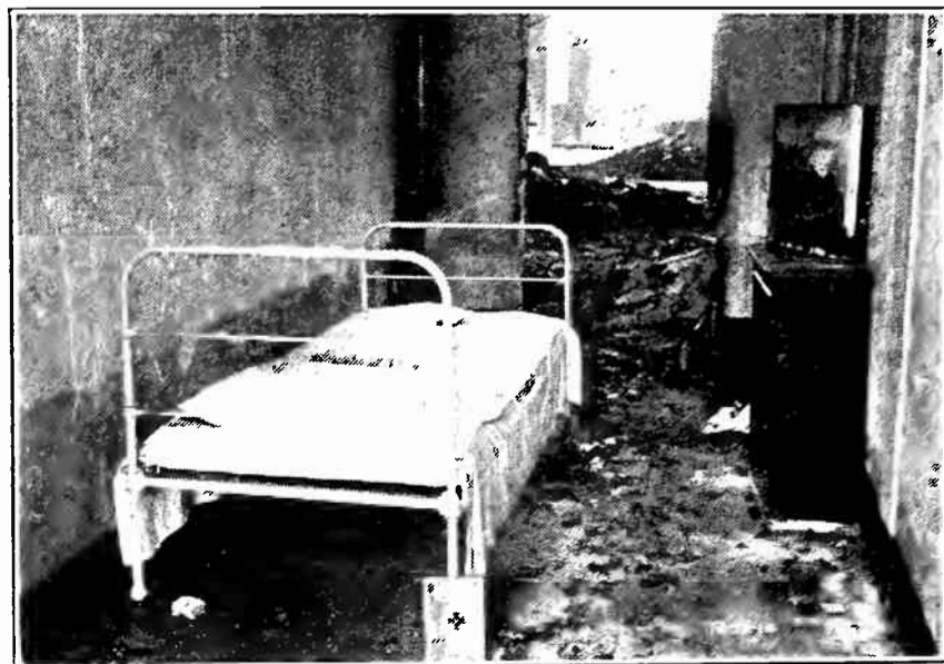
Although this "first aid to the injured" bed was on second floor, No. 24 Building, that was gutted, pieces of burnt wood were found on the floor near it, but the bed was untouched.
