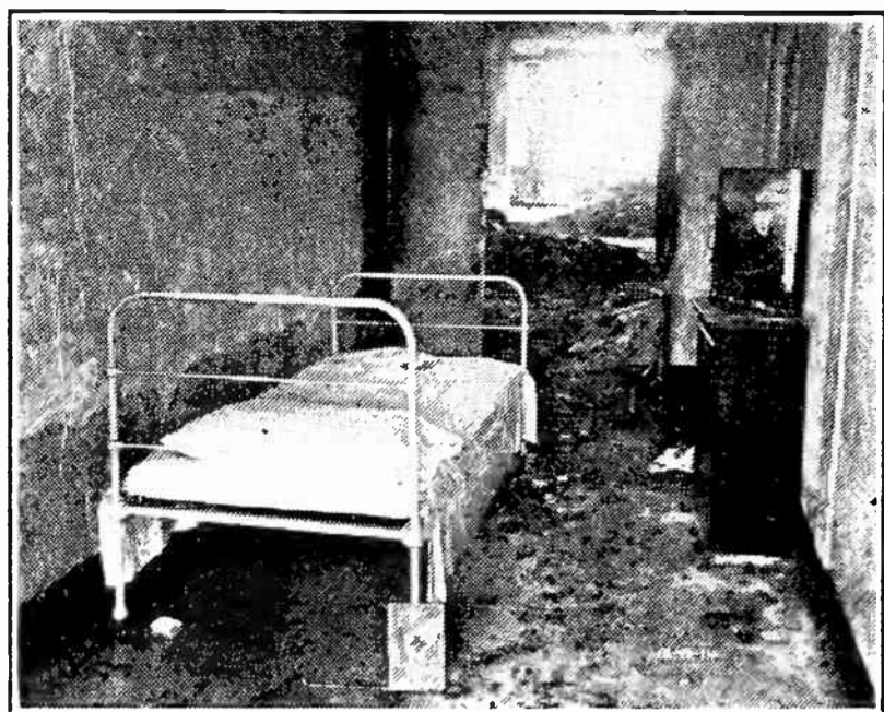
Although this "first aid to the injured" bed was on a floor that was gutted and pieces of burnt wood were found on the floor near it, the bed was untouched.
