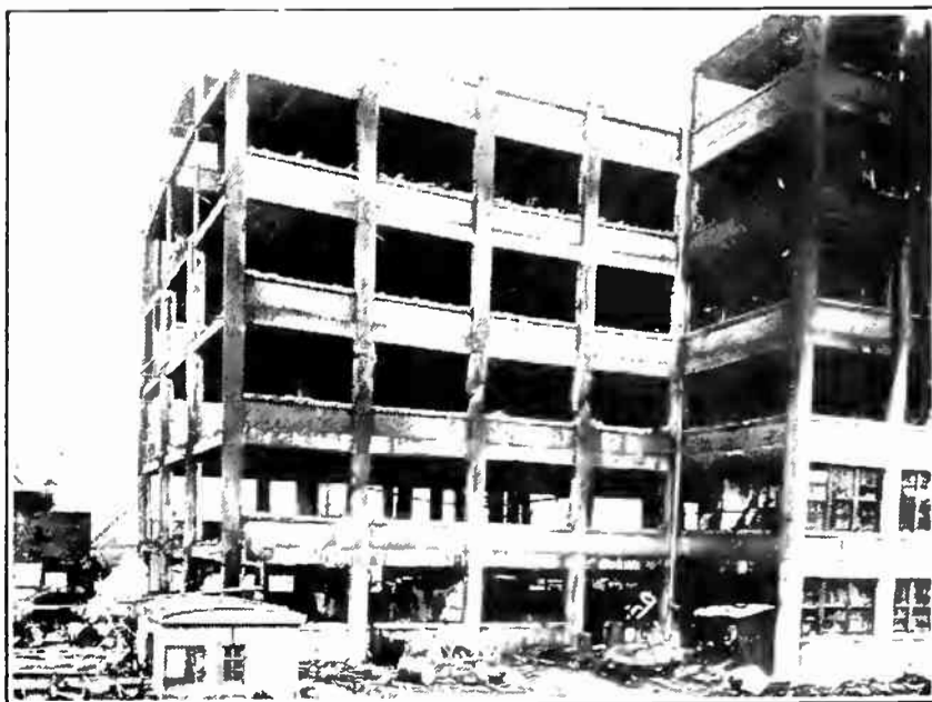
No. 24 Building—Northwest end—showing effect of fire and water on concrete. This end seriously damaged.
