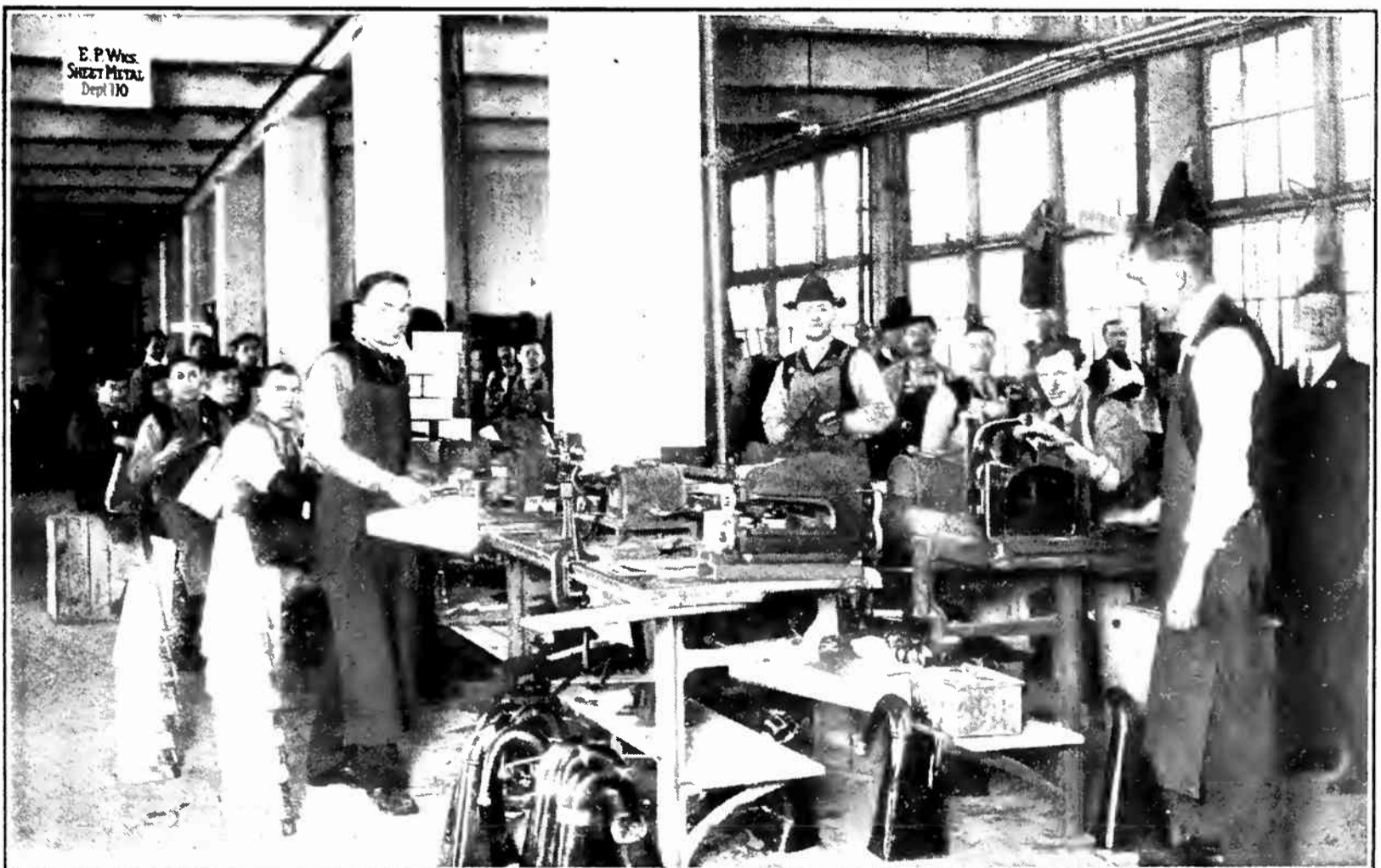
SHEET METAL DEPARTMENT, STORAGE BATTERY BUILDING
