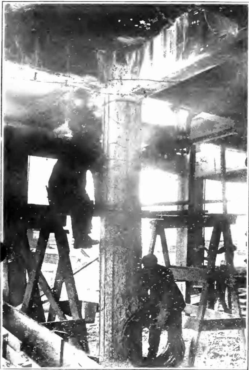
A CONCRETE COLUMN IN COURSE OF RECONSTRUCTION
