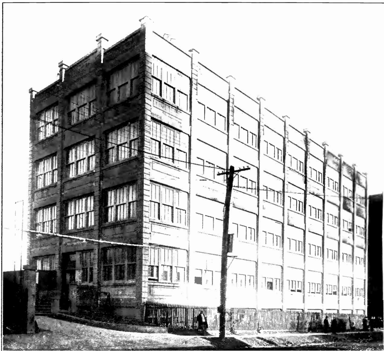
THE ADMINISTRATION BUILDING, SHOWING NEW STEEL WINDOW FRAMES AND SASH WITH WIRE-GLASS. ALMOST READY FOR RE-OCCUPANCY
