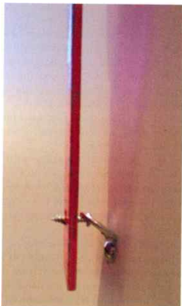
FIG. 1. I MARKED THE RING-HANGER SCREW LOCATIONS BY PRESSING AGAINST THE PANEL WITH THE RULER TAPED TO THE BACK.
