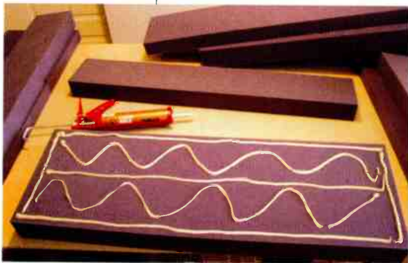
PRIMACOUSTIC'S ACOUSTIC PANELS ARE MADE BY ATTACHING FOAM PIECES TO A WALL OR BOARD WITH LIQUID NAILS, AS SHOWN HERE.
