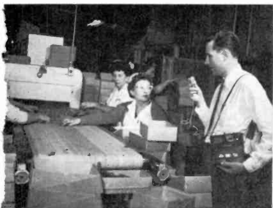
Left: checking production in a candy plant using an American Concertone TR 100 Transicorder. Center: quality control for the factory is expedited by on-the-spot use of the portable recorder. It is also useful in time and motion study work. Right: stockroom control and order filling are expedited by permitting purchasing and inventory personnel to record notes as stock is checked.
