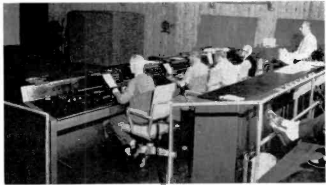
Seated at control console directly in front of screen, "mixers" (left to right) mix effects, mix dialogue, equalize music, and mix music, electronically juggling 96 sound tracks at a time.
