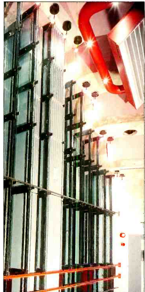
Real World's diffusing wall was one of the first to be modelled by computer
