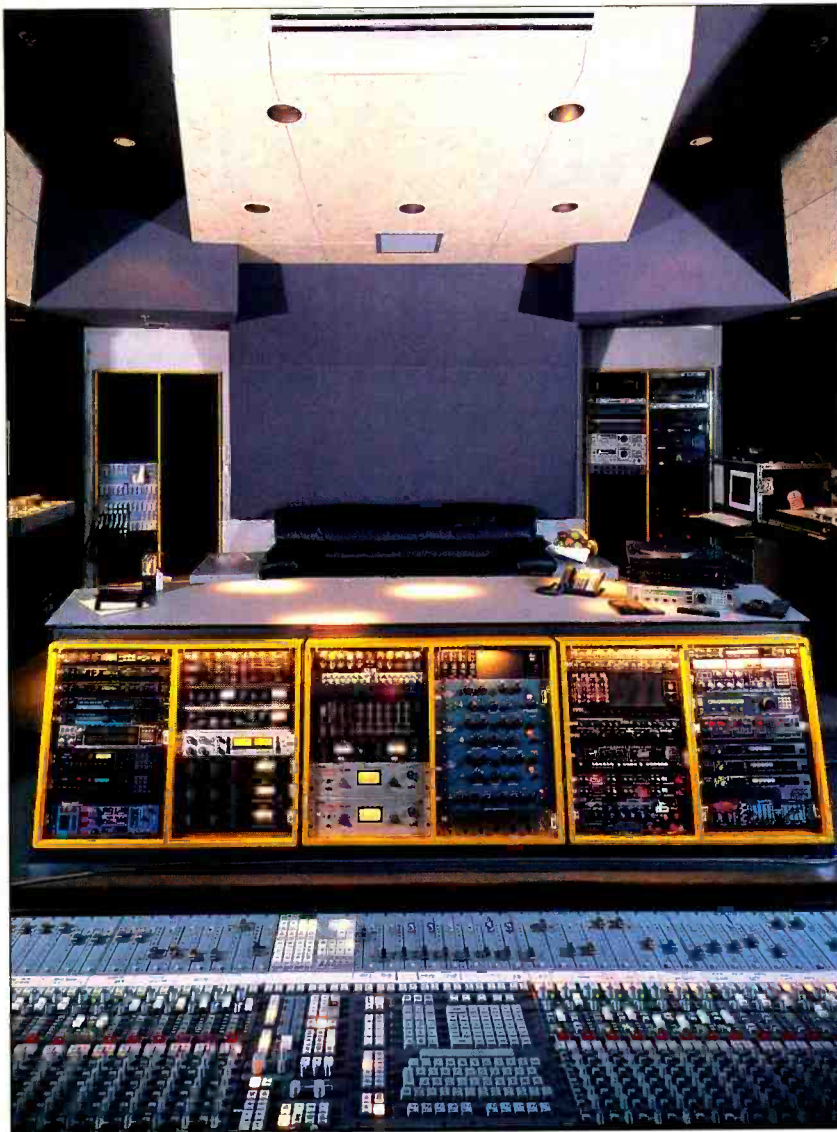
View of SSL1, showing outboard rack located behind SL-8000 G series console, and tape machine soffits
