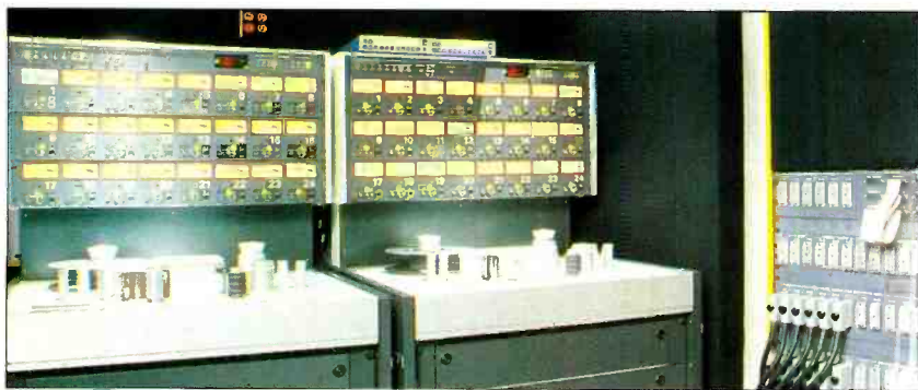
Multi-way connectors mounted beside each tape machine soffit allow analogue and digital transport to be swapped as the session dictates.
