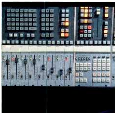
Part of the centre section
