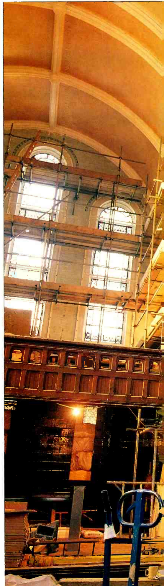
The restoration of the roof cost over £300,000 in just eradicating the rot, but has given Air room to improve the acoustic performance of the ceiling
