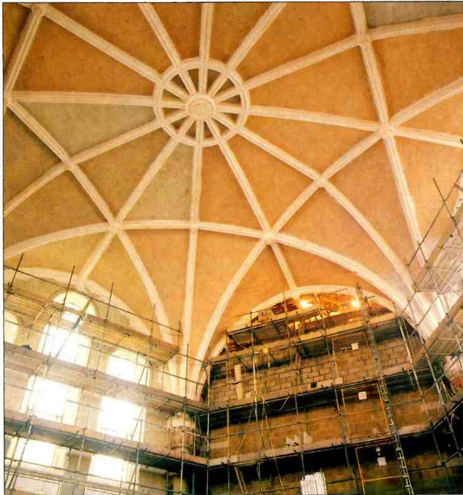
The restoration of the roof cost over £300,000 in just eradicating the rot, but has given Air room to improve the acoustic performance of the ceiling
