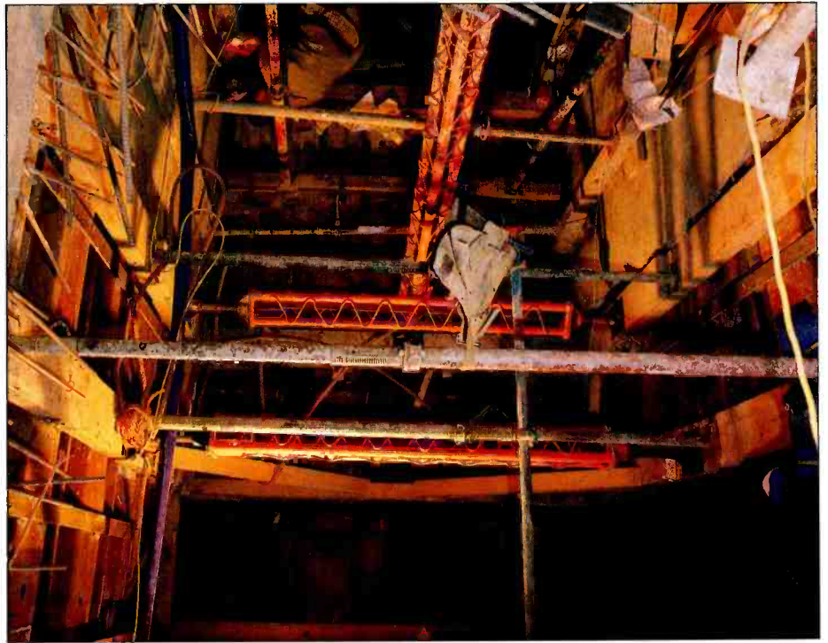
The basement is 5m deep, the lift shaft 7m
