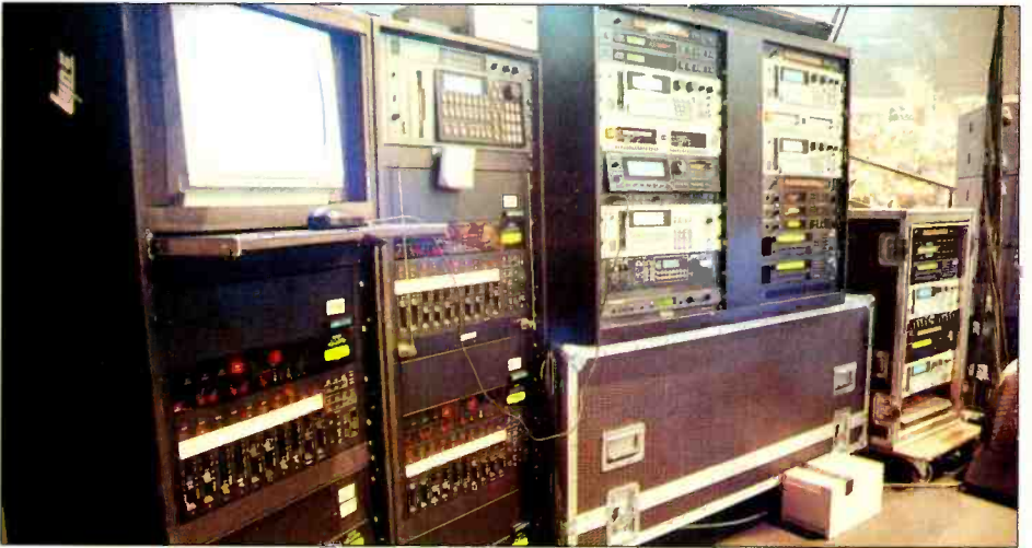
MIDI racks situated side of stage
