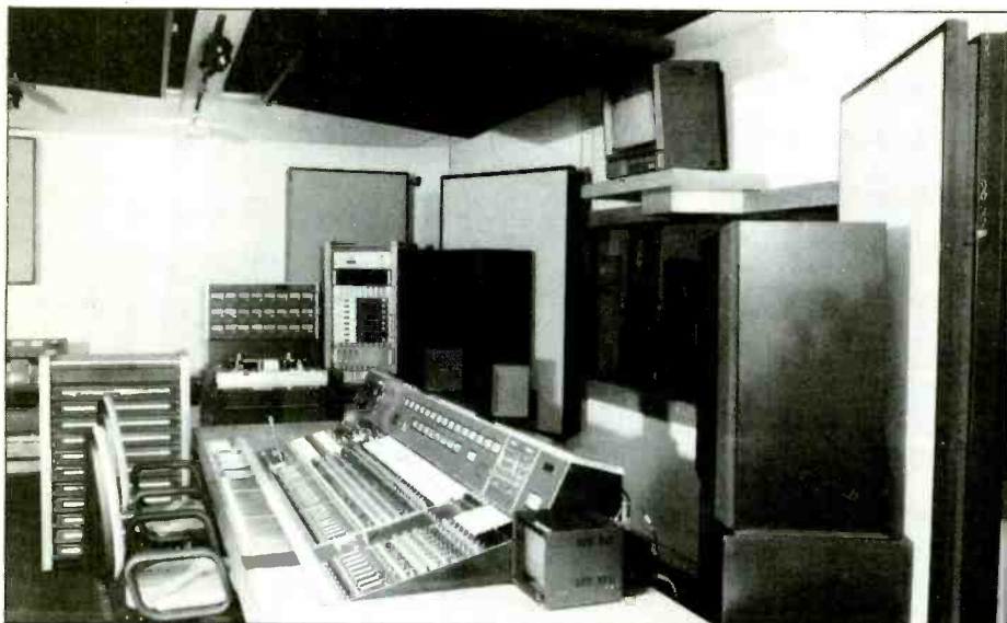
Black Box panels in Studio Two at CTS
