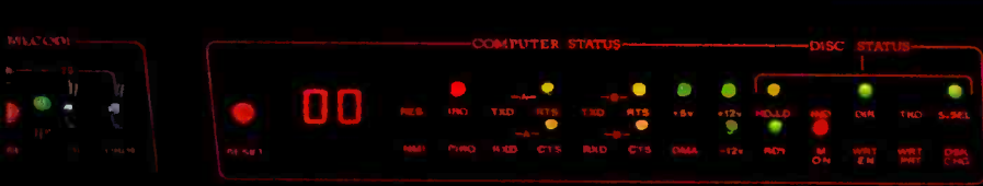
MASTERMIX MX 844 AUTOMATION COMPUTER
