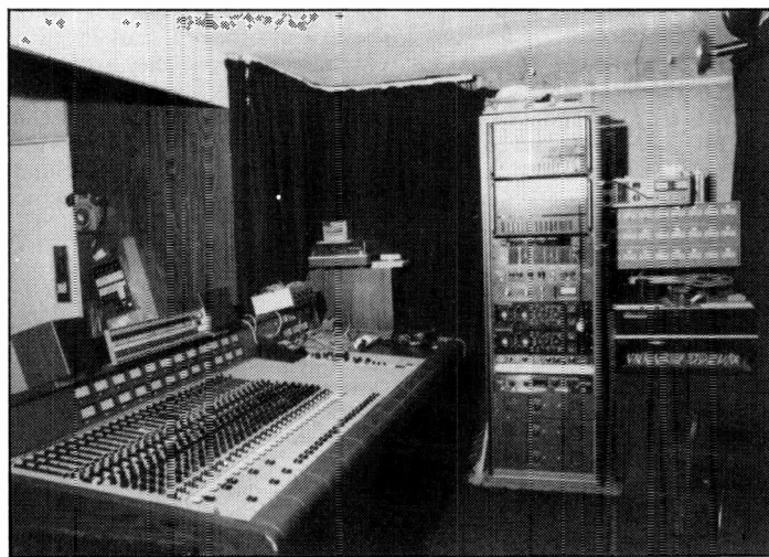
TW Studios with VCJH440 console. The payphone is hanging from the screw
