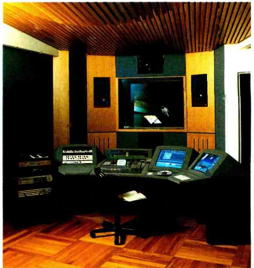
Italy: Vetriolo Studios, a 5.1 sound for picture facility in Milan, has recently installed a 16-track DSP Postation to sit with its Yamaha 02R and DynaudioAcoustics monitoring system. Vetriolo serves major music and postproduction clients including Honda, Volvo and Cointreau. The studio also posts independent films and documentaries, and authors and masters DVDs.
