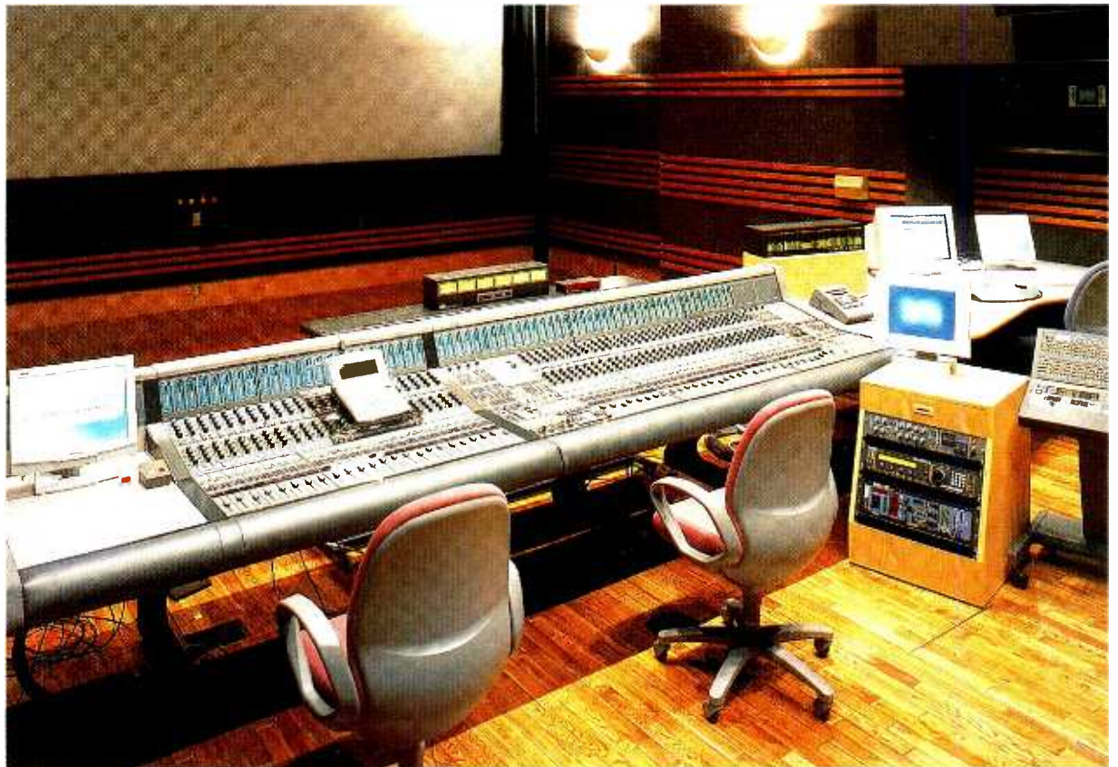
Japan: As part of its refurbishment, Tokyo TV has installed a AMS Neve Digital Film Console in its Studio 407. The 2-operator desk is lined up for a wide variety of television programmes and feature film work including IMAX, foreign films and multichannel work for special events. Executive VP and senior engineer Shuji Inoue commented: 'The DFC enables our engineers to concentrate on creative sound production and gives us a very efficient studio environment'.
