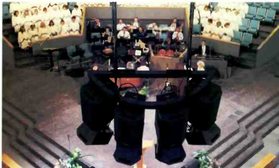
Center cluster array of AE-5s at the 2500 seat Valley Cathedral Worship Center, Phoenix
