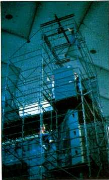
Figure 2. Audio Analysts technicians work with the sound reinforcement company's HDS full-range enclosures. One hundred forty-four of the speaker cabinets were used for the event, erected in triple tiers on the scaffold sound wings.
