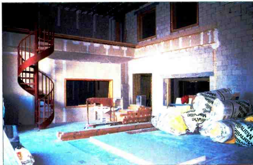
Photo 2. Studio V under construction.
