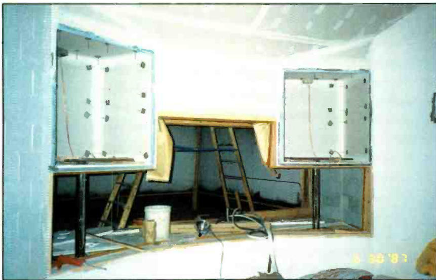
Front of Control Room B showing monitor pedestals under construction.
