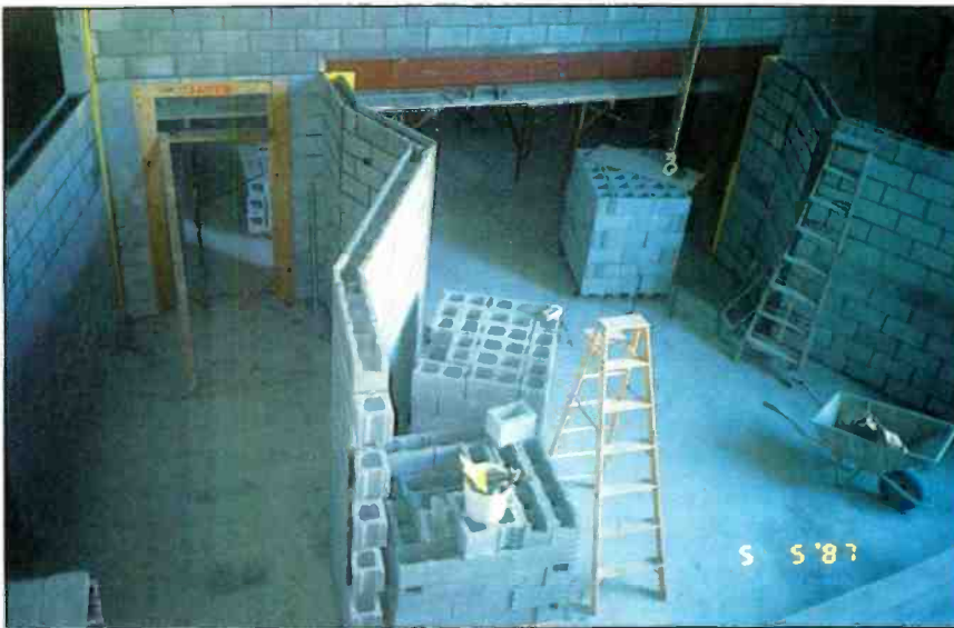
Construction phase of Control Room B.
