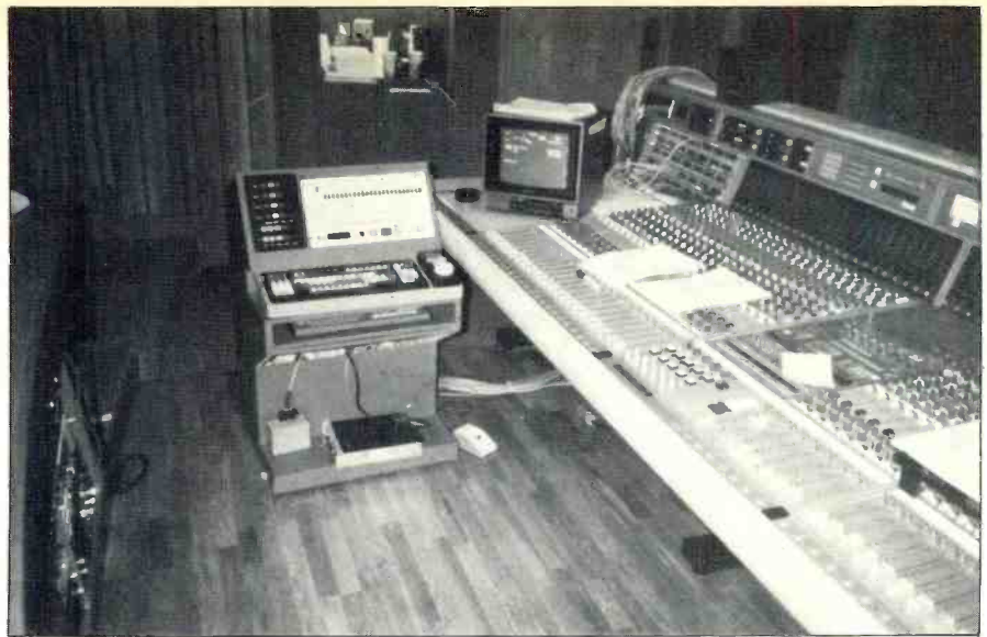
The Post Group’s new Studio A features a Neve 8128 console with NECAM 96 automation, seen here with the Otari MTR-90 remote and CMX synchronization controller.
