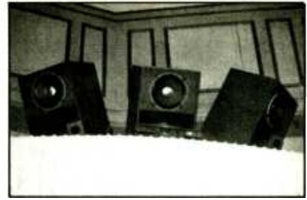
Figure 1: The Formal Ballroom's overhead cluster system is suspended above the proscenium stage, overlooking the dance floor.
