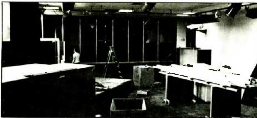
The Boathouse interior during studio construction . . .
