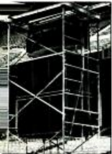
Figure 4: JM-10 in scaffold at Oakland Coliseum
