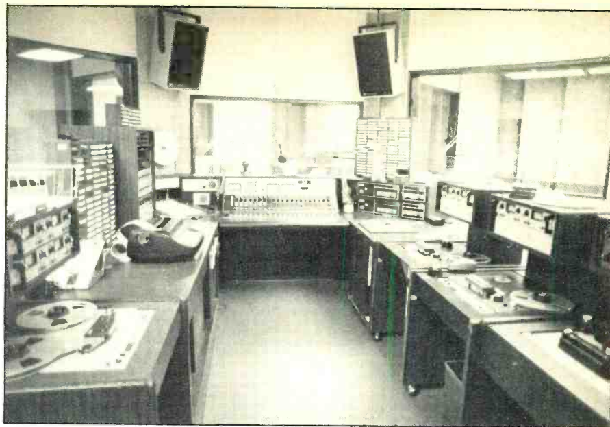
A MCI JH-110 four-track and Pacific Recorders stereo console form the basis of KFI's in-house production studio
