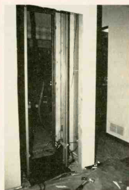
With the assistance of an architect, the Andersons broke through the wall separating the living room and den to create a space for their rack-mounted components—a Crown preamp, power amp, tuner, open-reel recorder, and speaker-switching module along
