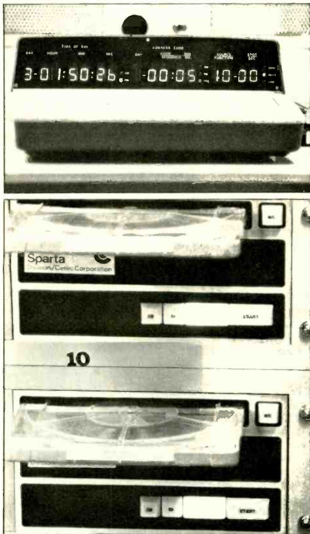
Top: Input terminal for programming automation equipment. "Time of day" is current; "address code," "source/function," and "spot/sec" determine what will be played and when.
