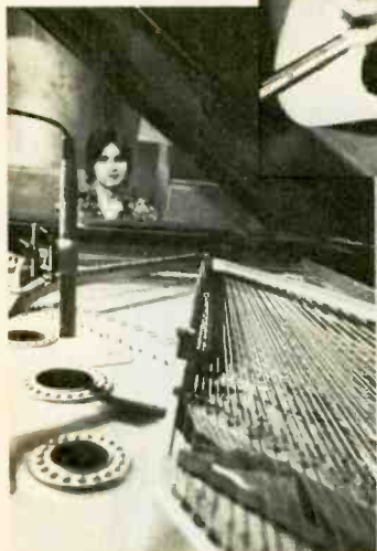
The microphone for Pete Romano's acoustic guitar is placed very close, to help minimize leakage from other instruments.
