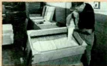
3. Sand is poured on, filtering slowly through small openings into panel cavities. Vibration machine eliminates air pockets, insures maximum compression.
