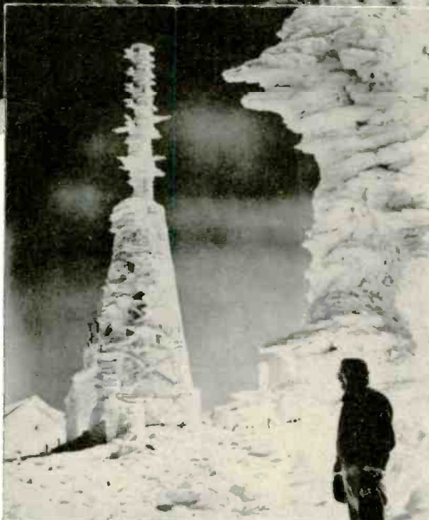
Close-up of broadcast facilities atop Mt. Washington, where the 310 tuner has performed steadily for over two years. This particular location is known as having "the world's worst weather." Note the extreme icing conditions.
