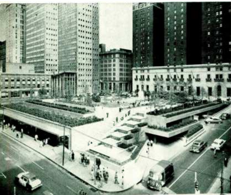
PITTSBURGH CHAMBER OF COMMERCE Mellon Square Park conceals a thousand-car parking garage.
