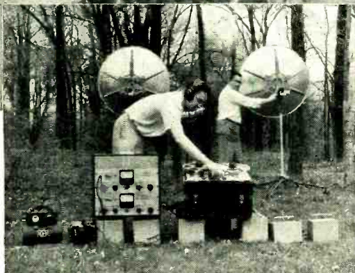
Robert Oakes Jordan and James C. Cunningham using two parabolic sound reflectors and two Shure Slendynes during an outdoor stereophonic recording session.
