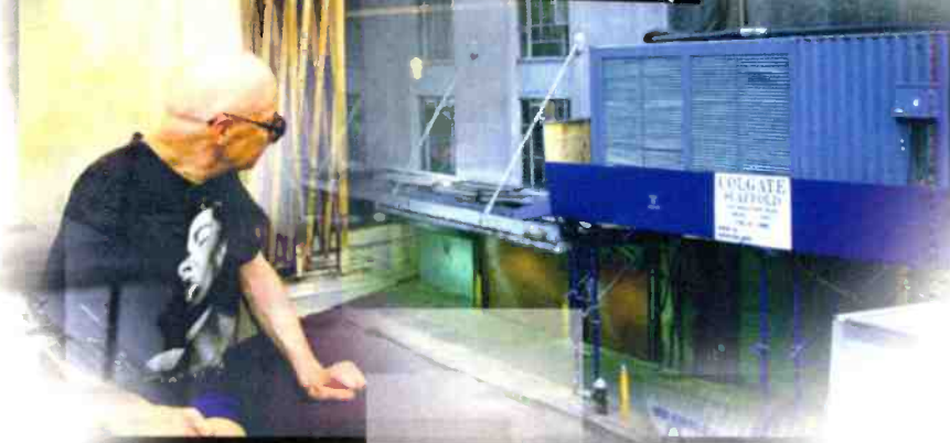
KALMEN (BELOW) AND PALTRIDGE HAVE FILED SEVERAL COMPLAINTS ABOUT THE MANHATTAN CENTER'S AIR CONDITIONER (RIGHT).
