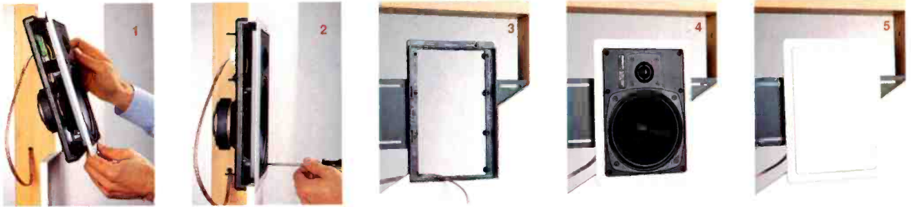
In-wall speakers, like this Boston Acoustics Model 381 ($500 a pair), are usually installed one of two ways. For existing walls, mounting tabs behind the baffle (or, in this case, a mounting frame) can be tightened
