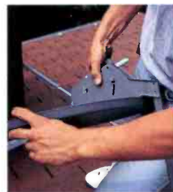
United Audio installer Jim Ephgrave heads for the roof with the 18-inch dish from RCA's Digital Satellite System (DSS) in hand. Before bolting the dish to its chimney-mounted support bracket, he adjusts its angle. Finally, he uses a portable DSS receiver/signal-strength meter to fine-tune the alignment for optimum signal reception.
