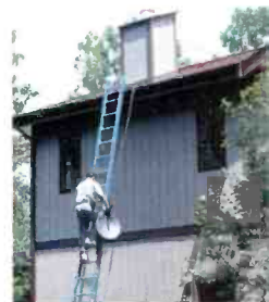
United Audio installer Jim Ephgrave heads for the roof with the 18-inch dish from RCA's Digital Satellite System (DSS) in hand. Before bolting the dish to its chimney-mounted support bracket, he adjusts its angle. Finally, he uses a portable DSS receiver/signal-strength meter to fine-tune the alignment for optimum signal reception.
