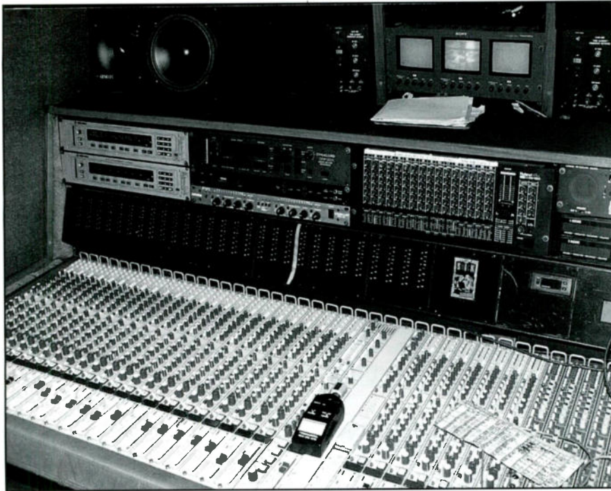
Figure 4. The dominant feature at the front of the room is the 36 channel Harrison MR-4 console.
