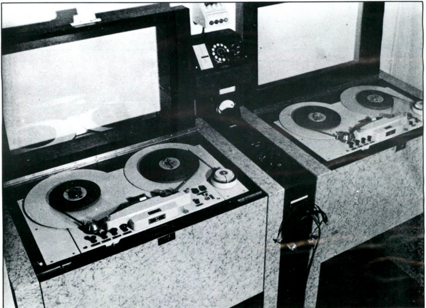
In 1938, the German radio or "Reichsrundfunk" became the first broadcaster in the world to adopt tape as its transcription and time-delay standard. Shown are AEG Magnetophon K-4 "HTS" AC-bias models at Radio Kiel, circa 1943.
