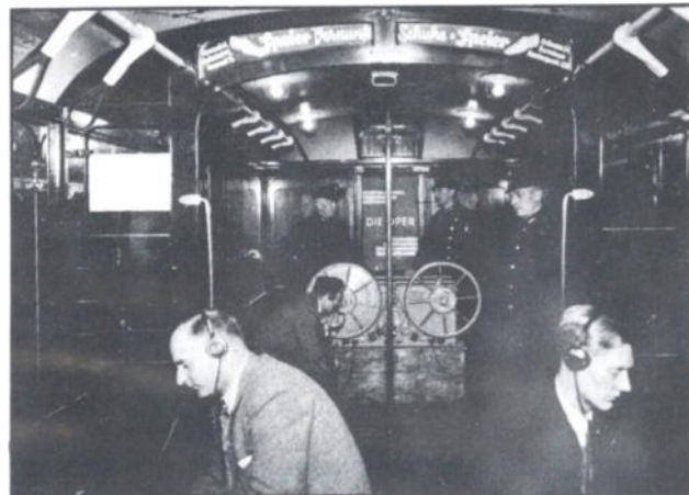
October, 1934 Sender Hamburg remote broadcast recording on a Hamburg commuter train, using the Lorenz Steeltone machine. (Photo courtesy of the Norddeutscher Rundfunk Archives, Hamburg, Germany.)
