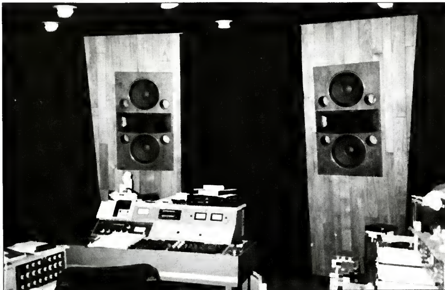
Figure 2. The Hidley Reference Design, one of two at the studio. Notice the vertical cone configuration with centered horn lens.
