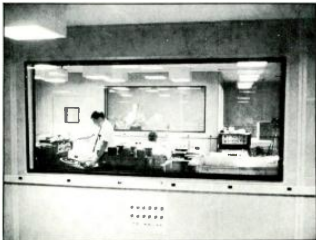
Figure 4. Proprietary windows in the recording studio of the U.S. Naval Training Devices Center, Orlando, Florida. (Courtesy Industrial Acoustics.)
