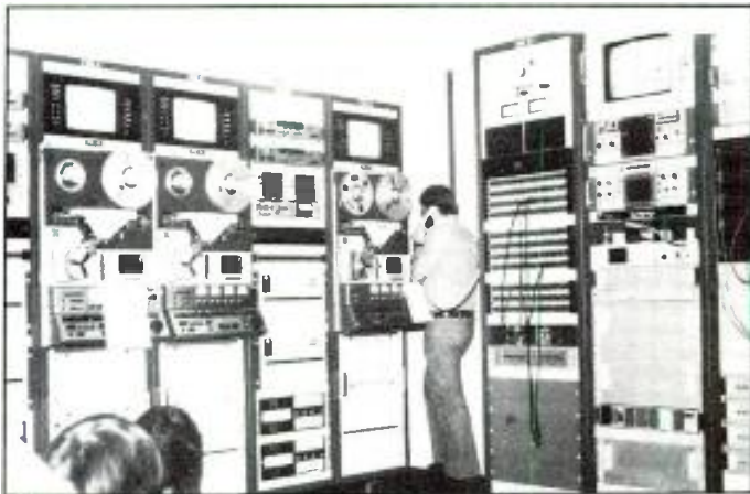
Figure 2. The SatCenter I control room.
