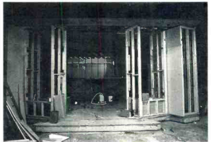
Facing the control room during framing and isolation stages.
