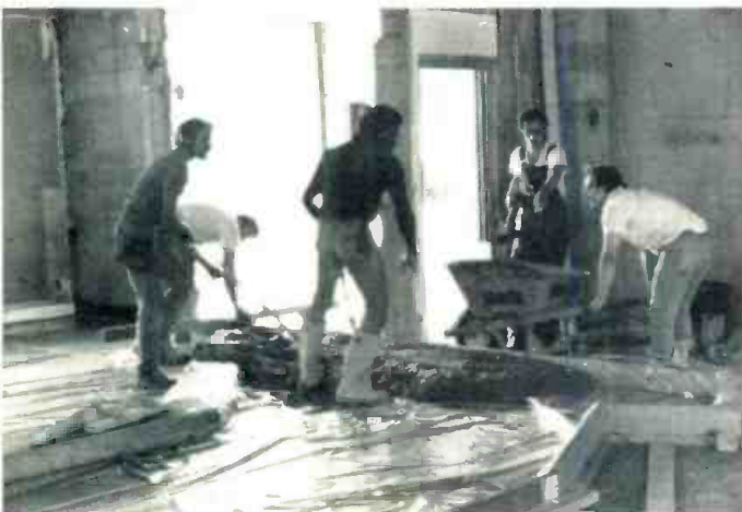
The concrete for the floated control room floor.
