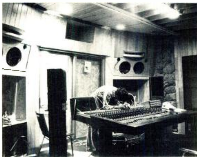
Interfacing during the finishing stages of the control room.
