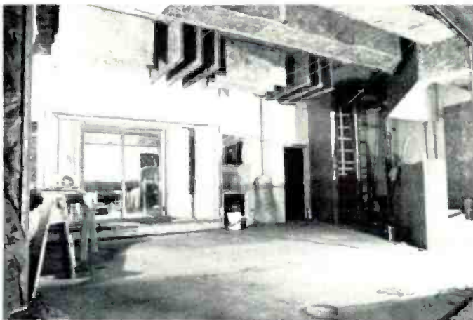
The studio under construction as viewed from the isolation room.
