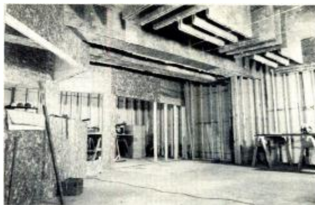
The studio under construction as viewed from the bass cage.
