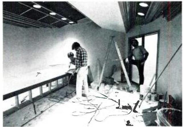
The studio control room under construction.
