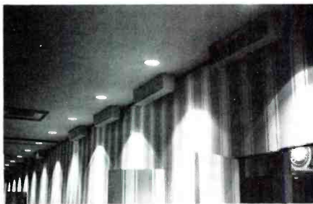
The line array of speakers in the foyer of the Grand Ballroom.
