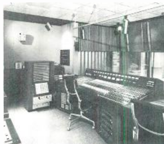
Figure 4. The main control room's custom-built board is behind a panoramic view into studio A.
