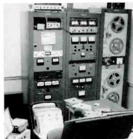
Figure 3. All in one room, WMNB-AM master control, remote transmitter and monitor racks, and background music tape decks.
