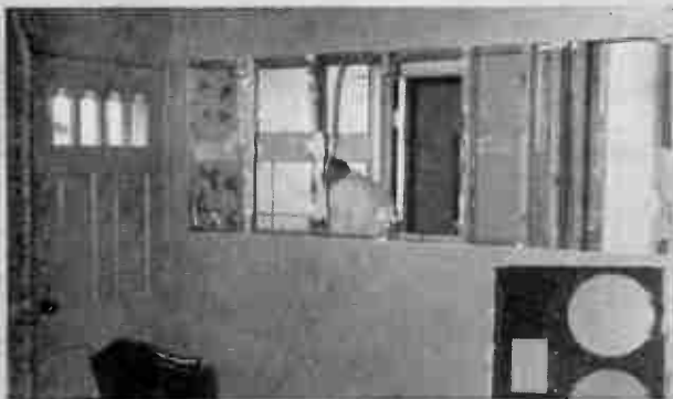
To make way for stereo, the old panel was removed, and the wall opening enlarged.
