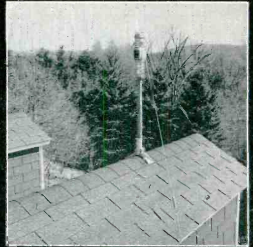
7 Over-all view of rotator and base. Guy-wire mount is most rigid of all.
