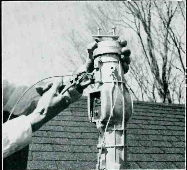
2 Rotator is bolted to one piece of mast, and guy wires, cut to proper length, fastened to rotator lugs.
