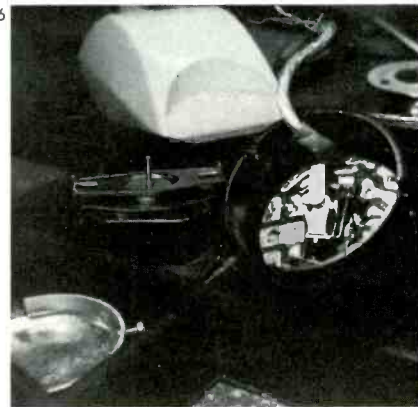
Fig. 4—Speed-change arrangements may include change of start capacitor and some complicated switching, as shown.
